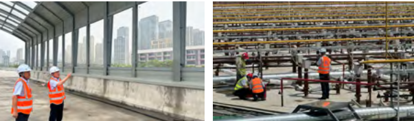
Environmental Protection Inspection on Construction Project Site
