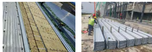
Installation Site of Roof Rock Wool
